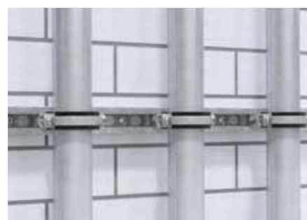
Mounting of water installations
