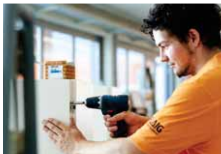
Installation of fittings on ends of boards
