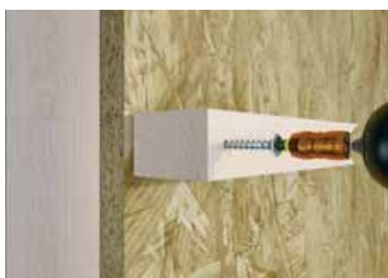
Mounting of installation level
