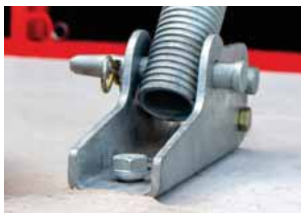
Installation of push-pull props/formwork
