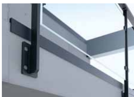
Fixing of railing
