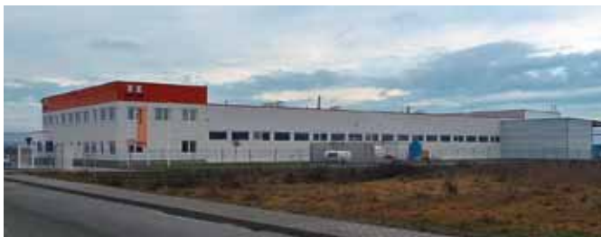
The plant in Câmpia Turzii, in Romania
