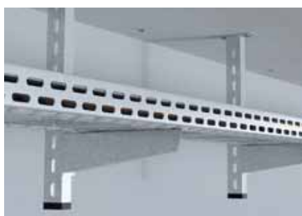
Fixing of cable ducts
